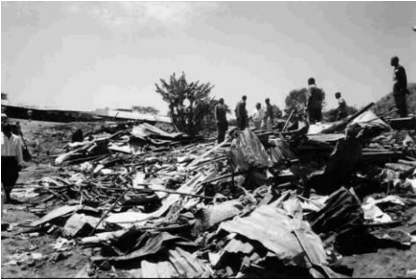
Demolition of Raila Village, 8 February 2004
